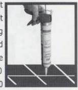
minutes). Tap the tile with the rubber mallet. Rotate the caulk gun to the other holes and inject until adhesive begins to come up through the holes. Clean excess with damp sponge or rag. When done, close the cartridge with cap provided.
