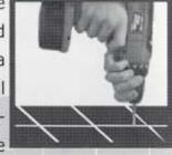
thickness of the tile. Drill 4 to 8 holes around the loose tile. Be careful not to drill into the tile.
